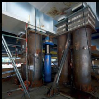
**605 tons locknut cylinders**
