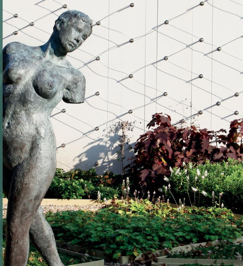
The green line posts individually take loads up to 100 kg and should be used with a maximum distance of one meter.
