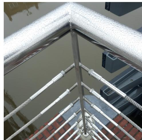
Stainless steel is a wonderful material, and treated properly, it will stay bright and stainless forever. Sadly, natural saltwater is one of the most aggressive and corrosive media towards stainless steel, and even the "acid resistant" 316L class requires a bit of maintenance in order to stay stainless.
